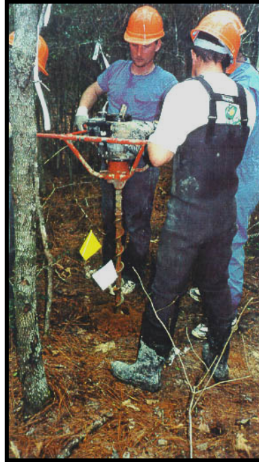
Use of hand portable drills to drill mini-hole patterns that are used in some seismic surveys minimizes vegetation cutting and soil disturbance.
