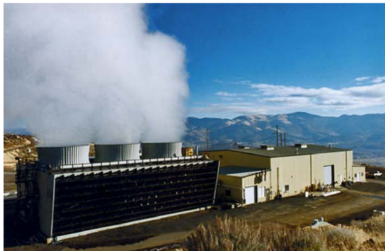
This geothermal steam power plant in Steamboat Springs, Nevada, emits mostly water vapor.
