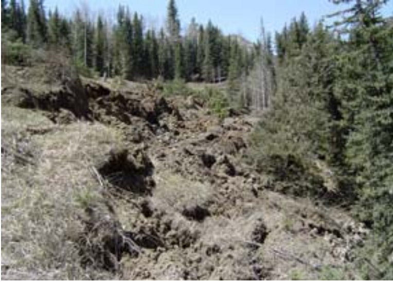
Same area as previous photo, showing actively sliding area below the old road and leaning trees that have been tilted as a result of slide movement.
