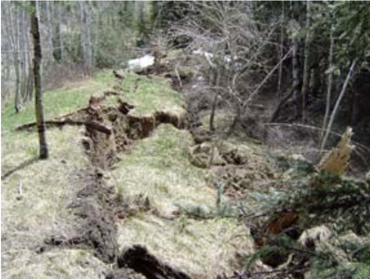
Cracking and shifting of the ground above the old road.
