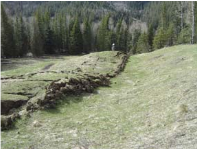
Same area as previous two photos. The area on the left of the crack where the person is standing is moving downhill and vertically up. The area on the right of the crack has not moved.
