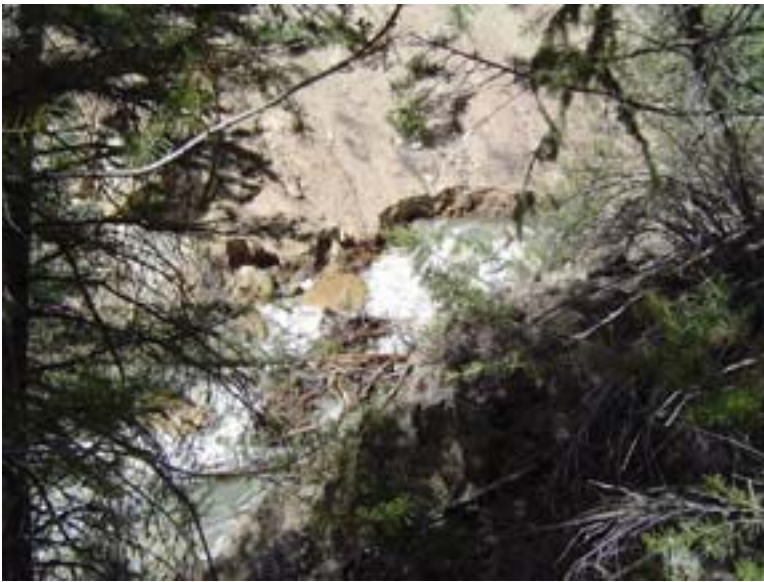
View of the East Fork of the San Juan River showing erosion of the stream bank across the river from the active slide. Photo also shows woody debris (trees) that have slid into the river and been washed downstream.
