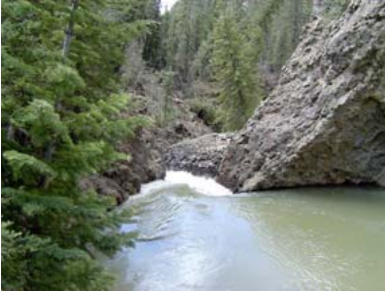
The slide is moving down the slope from the left of the photo and encroaching on the East Fork of the San Juan River.
