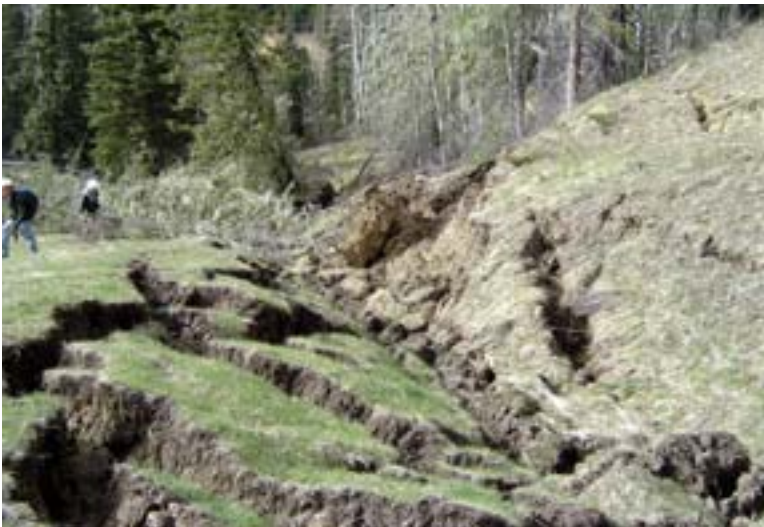
Cracking and shifting of the ground above the old road. The photo is looking downhill at the eastern edge of the active slide.
