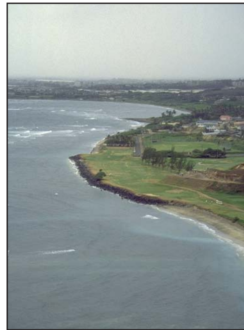
Seawalls line much of the Wailuku waterfront to protect urban and commercial infrastructure as well as county and municipal lands such as the Waiehu Municipal Golf Course at Waiehu.
