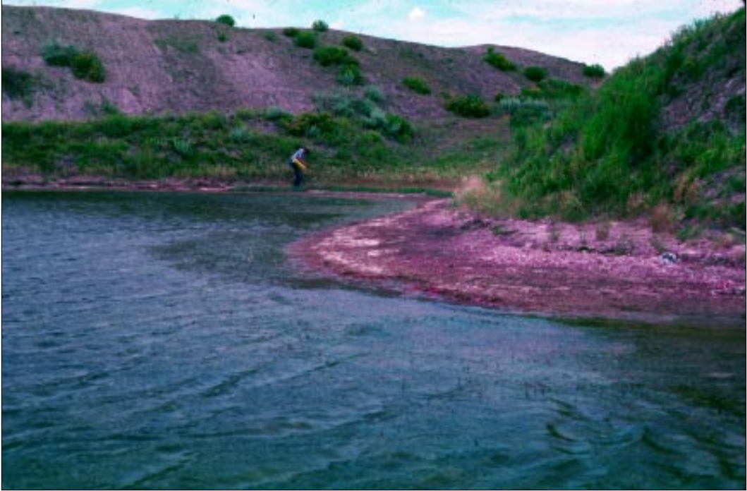
Figure 6. Basin slope is a major factor controlling the development of wetland vegetation in constructed wetlands. Interacting with fluctuating water levels, basin slope influences wetland plant community development by regulating water depth and permanence within zones of wetland plant establishment. (Photo by Rich Olson)
