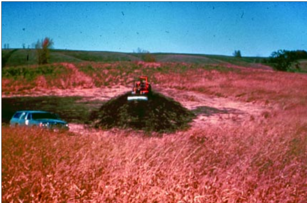
Figure 14. Islands should be developed during construction by mounding excavated basin material with bulldozers, draglines, scrapers, or dredgers. Linear-shaped islands with irregular shoreline contours, approximately 50 feet wide and 200 feet long with gradually sloped shorelines, are ideal for waterfowl use. (Photo by Rena Baldwin)
