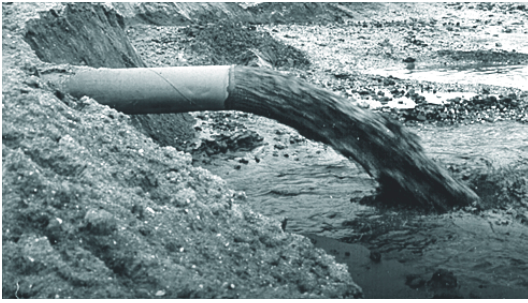
A total of 180,000 cubic yards of sediment was dredged from Pine Lakes as part of a comprehensive project that targeted watershed protection and lake renovation.
