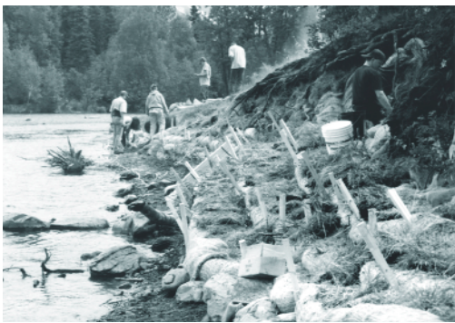
Casey and Ivy (right) work on an undercut bank as Dean Davidson, Assistant Director, and Vera Group instruct youth on proper use of erosion mat.
