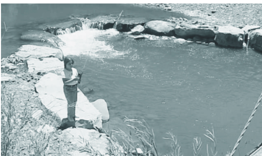
Aquatic habitat was improved by adding a drop structure. The pool in this area is 7 feet deep and supports trout.
