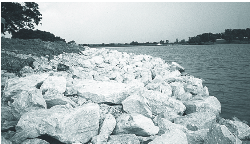
Streambank stabilization was a key component used to reduce sediment delivery at Pine Lakes.
