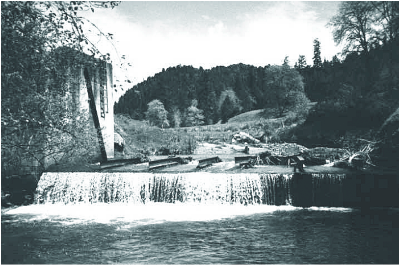
The concrete apron of the diversion structure spanned the creek with a 2-foot outfall at summer flows. This barrier prevented fish from reaching 10 miles of stream habitat.
