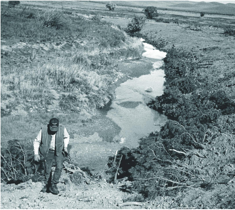
After sloping and revetments, outdoor classes were held and willows were planted at the site.
