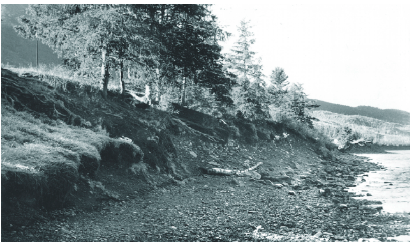
The Sanctuary Project is one of many efforts to restore eroded streambanks like this one at the mouth of the Russian River.
