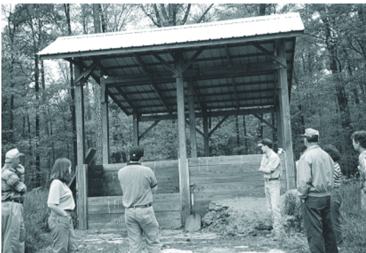
Project partners built a two-cell composter on the Johnson Poultry Farm to reduce nutrients from poultry waste runoff.
