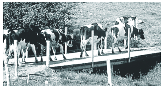
A bridge was constructed to allow cows to cross the stream without contributing to streambank erosion.
