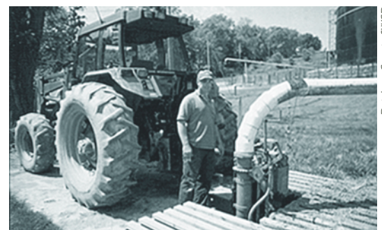
Peter Coon prepares to power up the primary pumping station to the farm's new waste storage facility.
