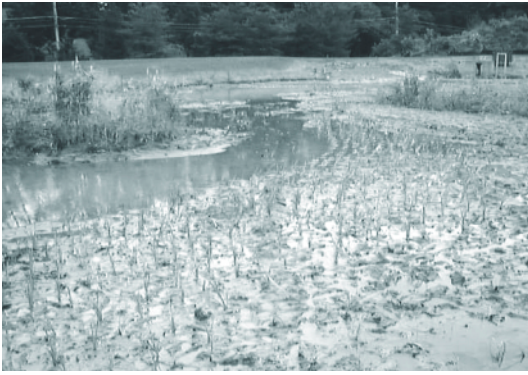
A meandering channel was designed to reduce flow velocity and allow particles to settle out.
