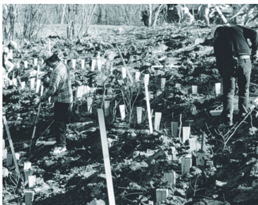
Willows were planted along the restoration site to provide long-term stability.
