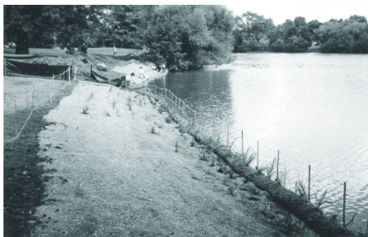
A coconut fiber roll and soil erosion blanket protected the bank until vegetation was established.
