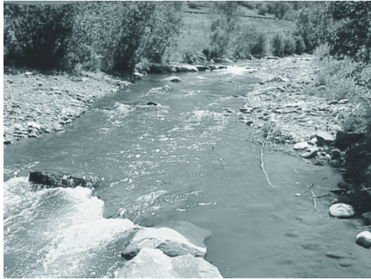
The J-hook in the foreground is typical of the structures installed in the river. It directs stream flow toward the thalweg and away from the banks.
