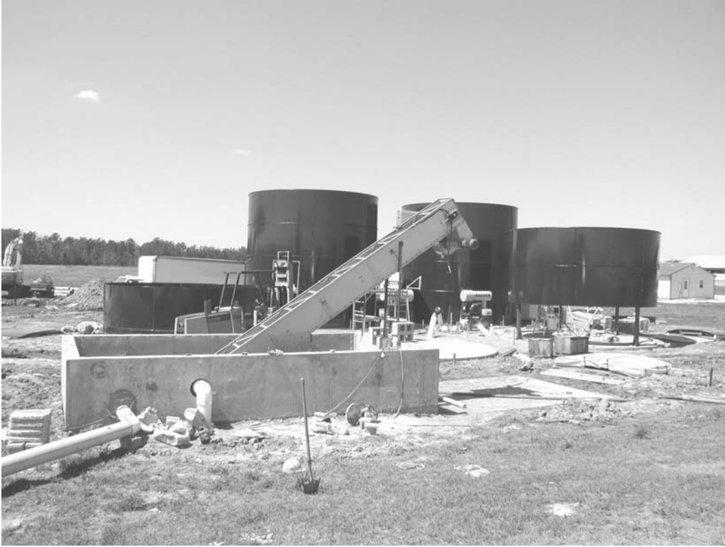
Figure 15. EKOKAN Solids Separation System
