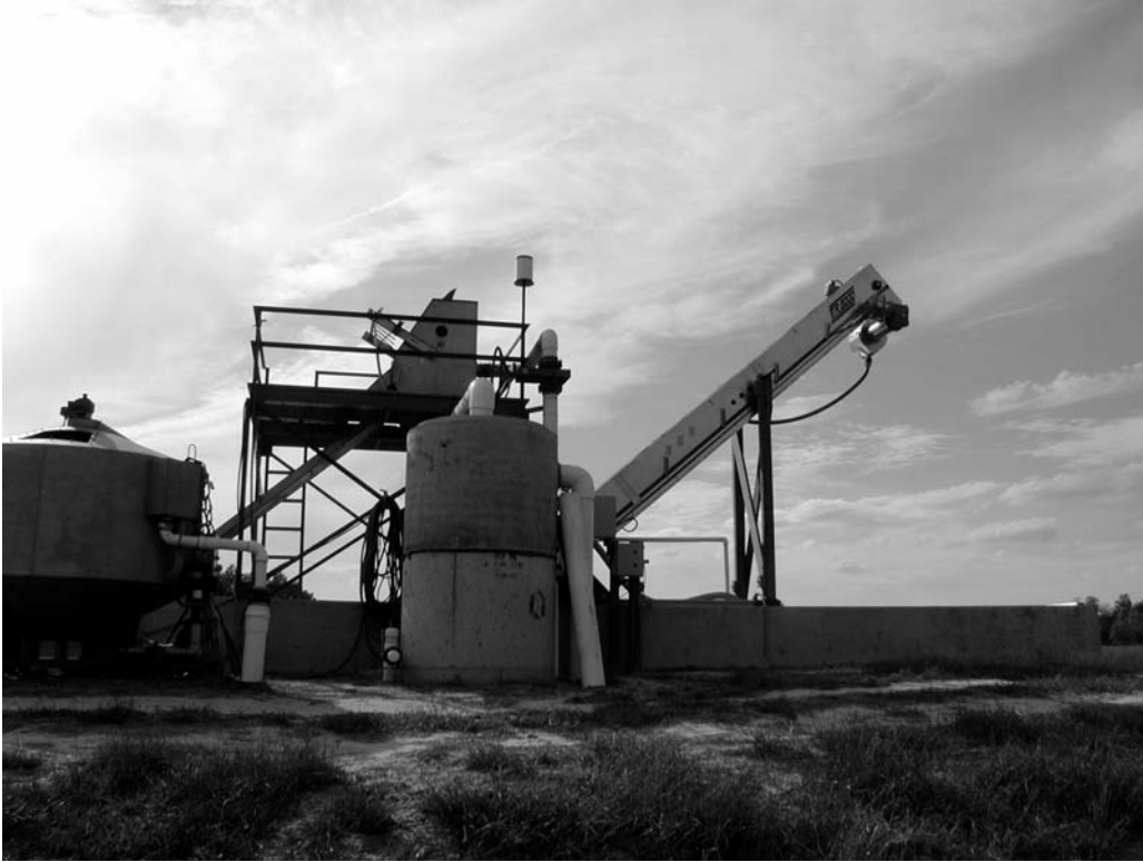
Figure 11. Solids Separation Equipment
