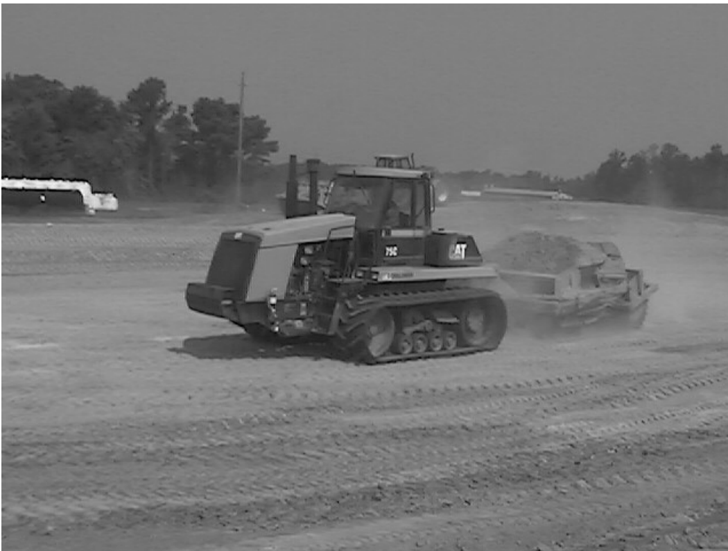
Figure 8. Excavation of the Constructed Wetland Cells
