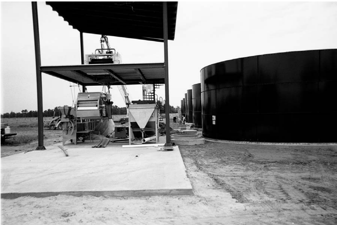
Figure 22. Processing Building and Above Ground Tanks
