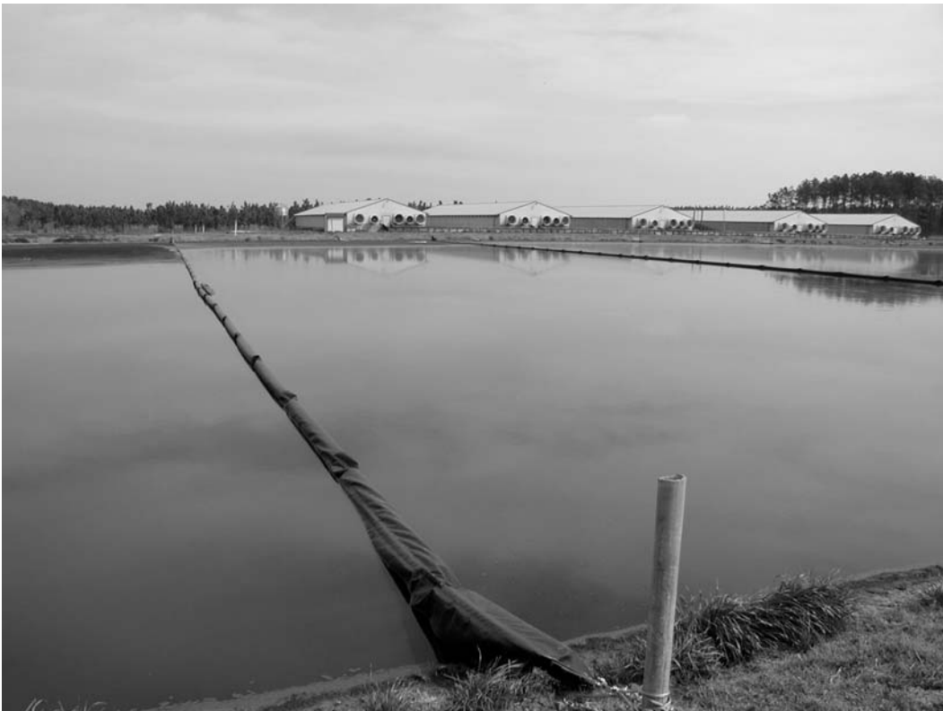
Figure 14. Curtain Baffle in Existing Anaerobic Lagoon
