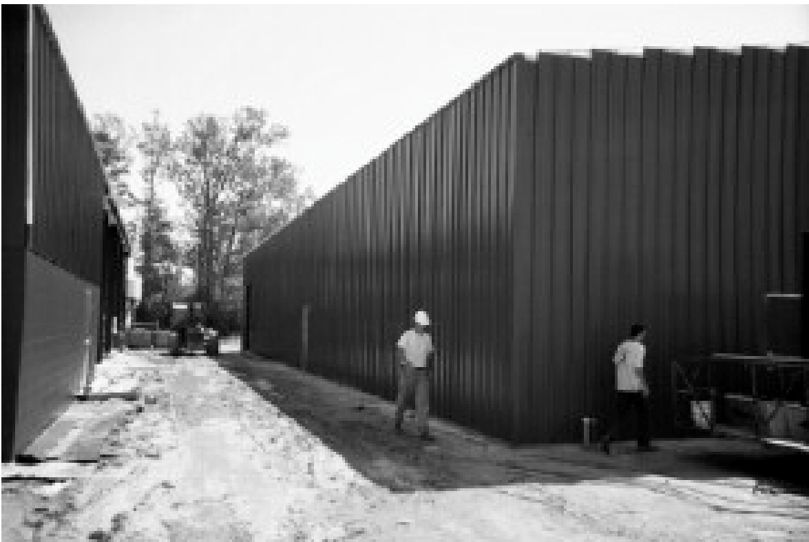
Figure 24. Solids Processing Facility
