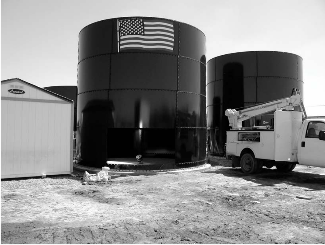
Figure 13. Completed EKOKAN System
