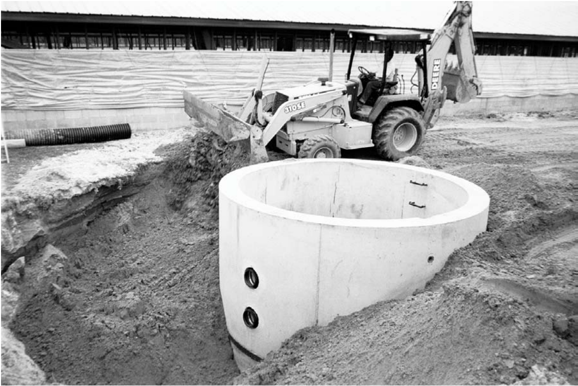
Figure 23. Concrete Store Tank
