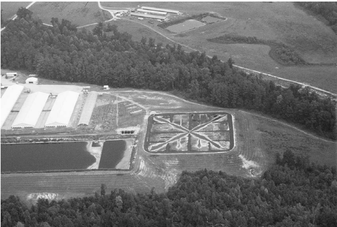
Figure 2. Aerial View of Ambient Temperature Anaerobic Digester & Nitrification System
