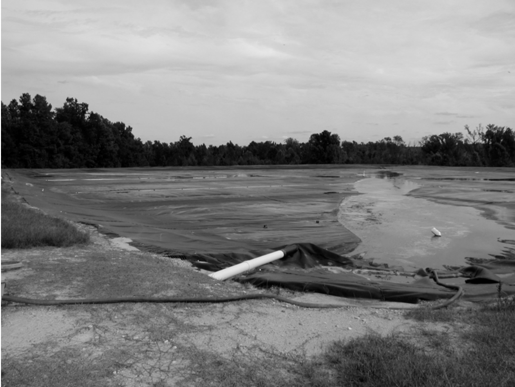
Figure 3. Covered Ambient Temperature Anaerobic Digester
