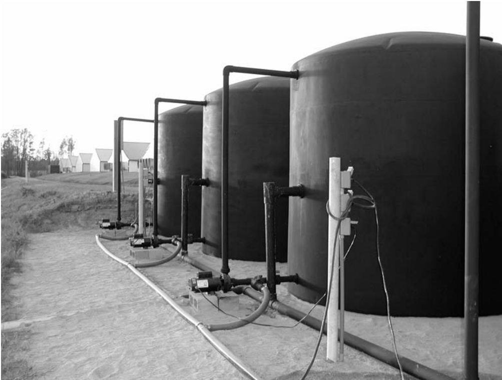
Figure 5. Nitrification Tanks
