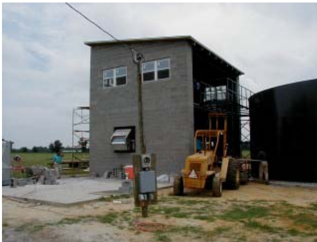
Figure 2. Solids-Liquid Separation Building at Production Farm (Goshen Ridge)
