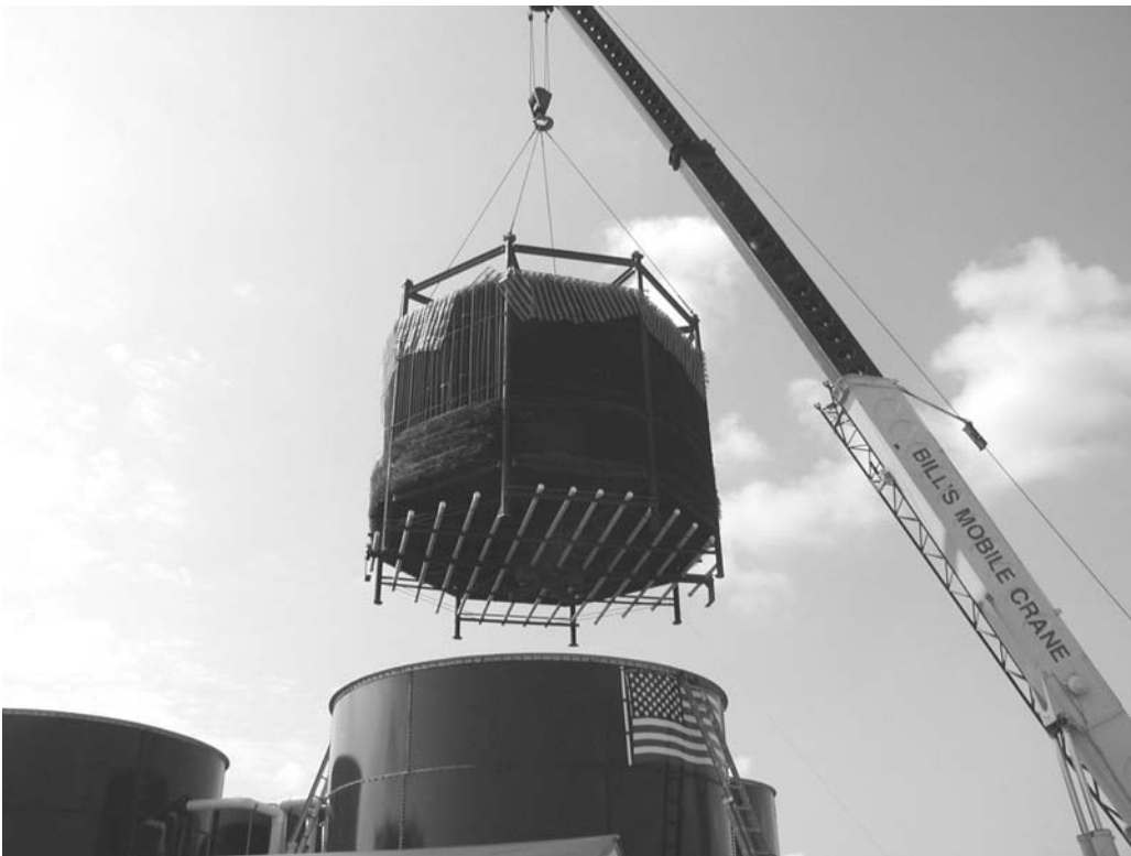
Figure 18. Installation of Filter Media
