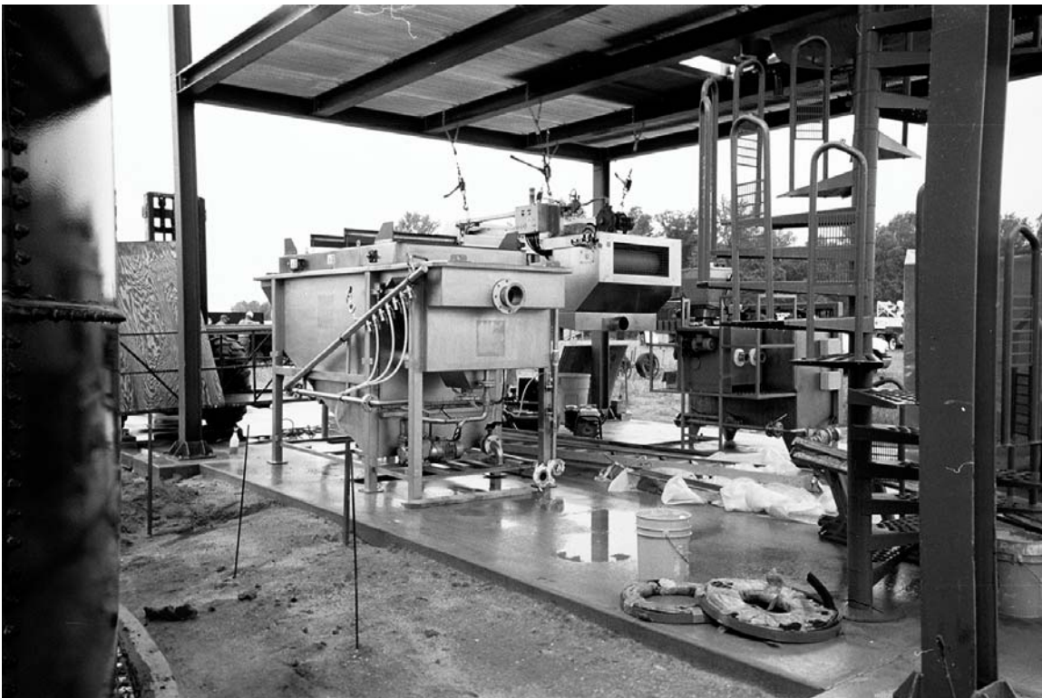
Figure 20. Dissolved Air Flotation Unit
