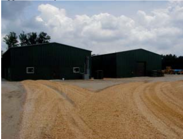
Figure 1: Constructed Solids Processing Facility at Hickory Grove Rd. Farm
