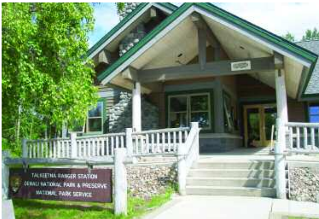
National Park Service photo
