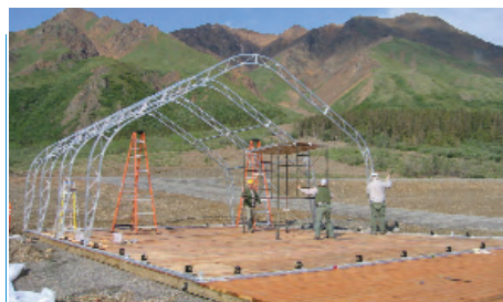
In June park staff erected a large weatherport to serve as an interim visitor contact station at the Toklat Rest Stop while the new Eielson Visitor Center is being constructed. The temporary facility includes exhibits and a sales area for the park's cooperating association.
