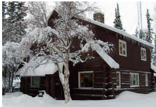
Denali National Park and Preserve Headquarters: Operating facilities in Alaska’s harsh subarctic environment contributes to high expenditures in Facilities Operations.
