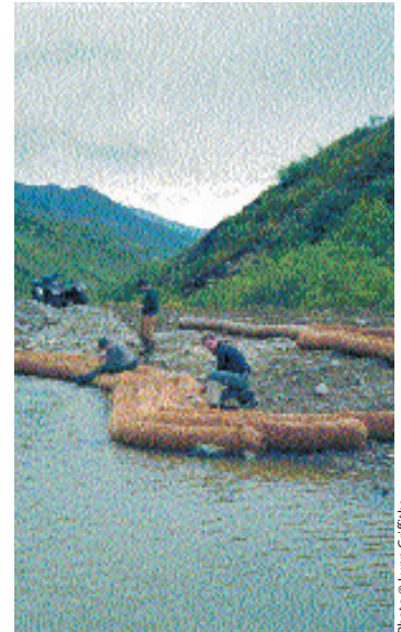
Coconut fiber logs are positioned to stabilize the banks of Caribou Creek
