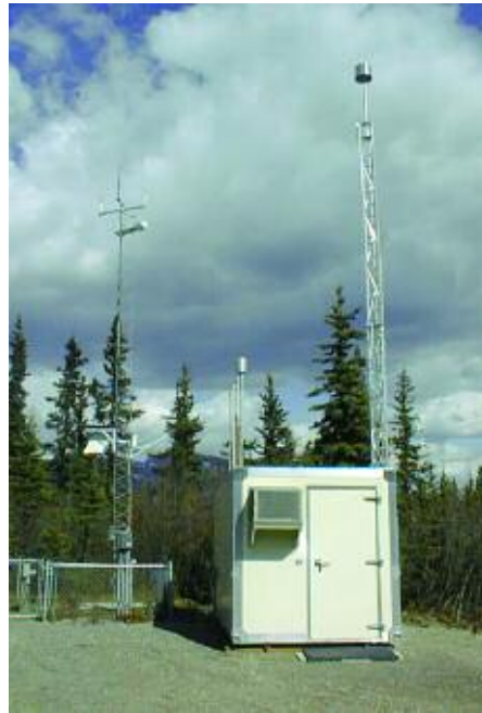
Air quality monitoring shelter near park headquarters.
