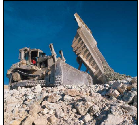
(Above is a picture of a bulldozer at a construction site.)
