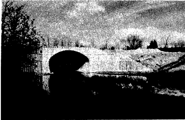
Figure VI-10--Culvert with metal headwall and wingwalls (ARMCO).
