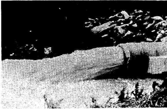
Figure I-11--Culvert flowing full (no tailwater at outlet end).
