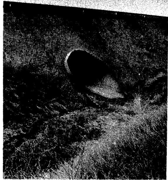
Figure VI-33--Unanchored mitered end.
