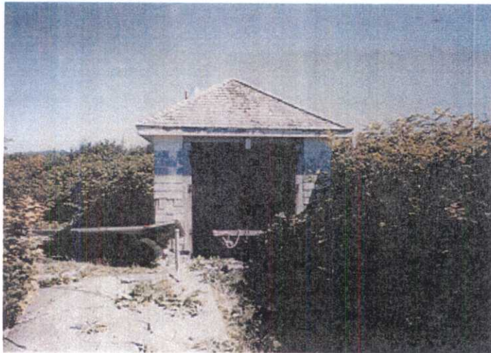
Photograph 7: Tram Car Shed.
