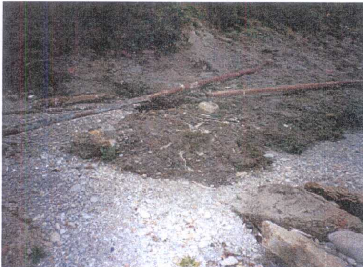
Photograph 13: Debris on Beach Below Garbage Dump Area.
