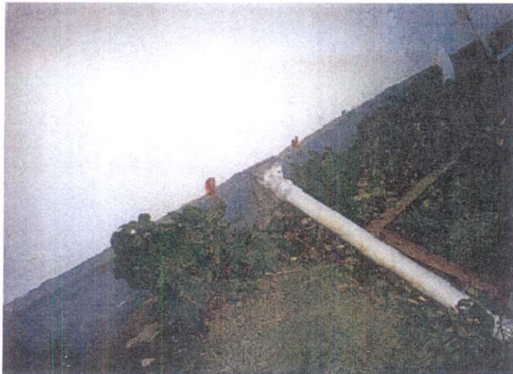
Photograph 2: Drain Line in Back of Fog Signal Building.
