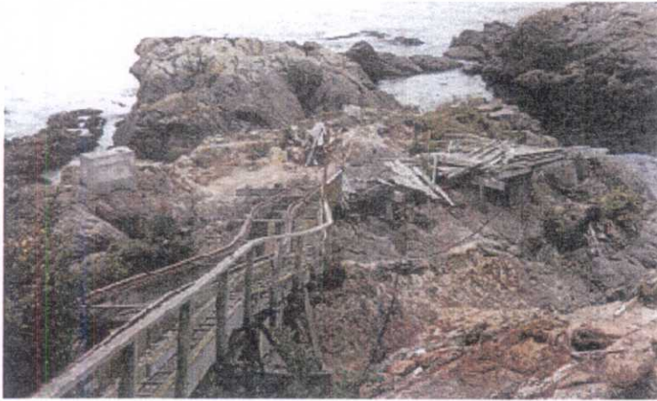
Photograph 15: Landing Dock Area.
