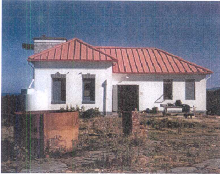
Photograph 1: Fog Signal Building.
