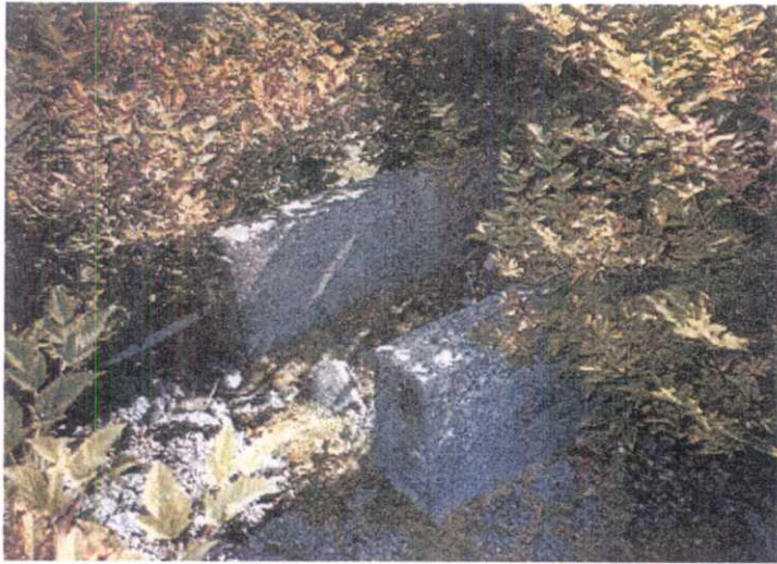
Photograph 9: Concrete Footings for Former AST.
