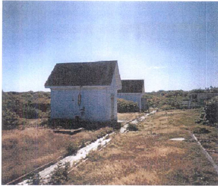
Photograph 3: Former AST Foundations, Paint Locker and Oil House (in background).
