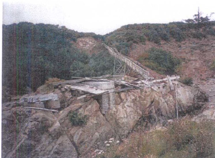
Photograph 14: Landing Dock Area.
