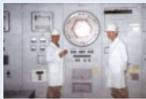
Control center panels for the BN-350 Breeder Reactor at Akhtau, Kazakhstan
