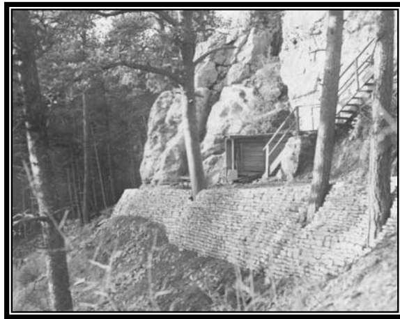
Figure 7-5. The new trail and stone terraced embankment to the Jewel Cave entrance was completed by the Civilian Conservation Corps in 1935 before the earlier wooden steps descending over the rocky ridge above the cave opening (to the right of the entrance) were removed. Courtesy of Mount Rushmore National Memorial (JECA 2797).
