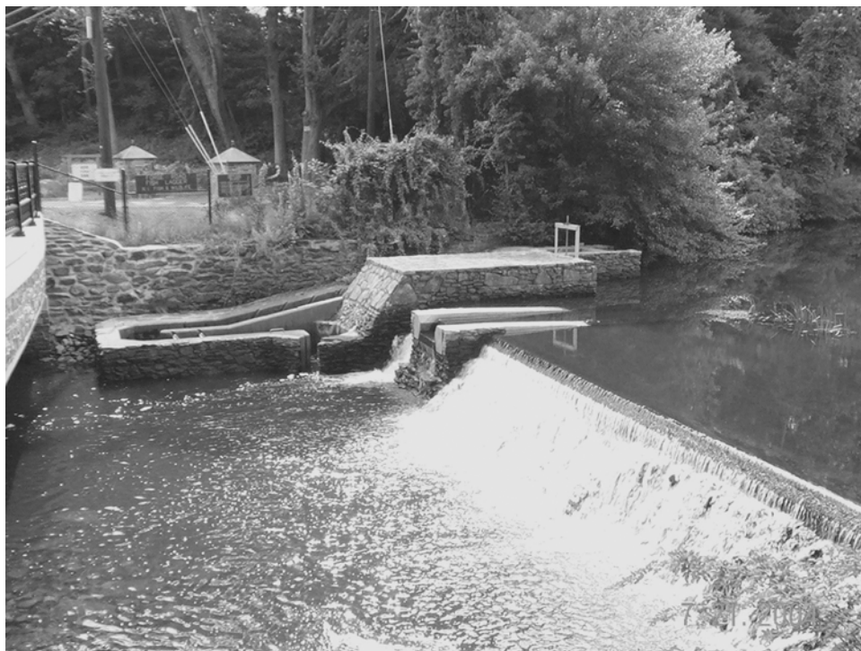
Fish ladder at dam near USGS streamflow gaging station on Hunt River near East Greenwich, RI, 0111700.
