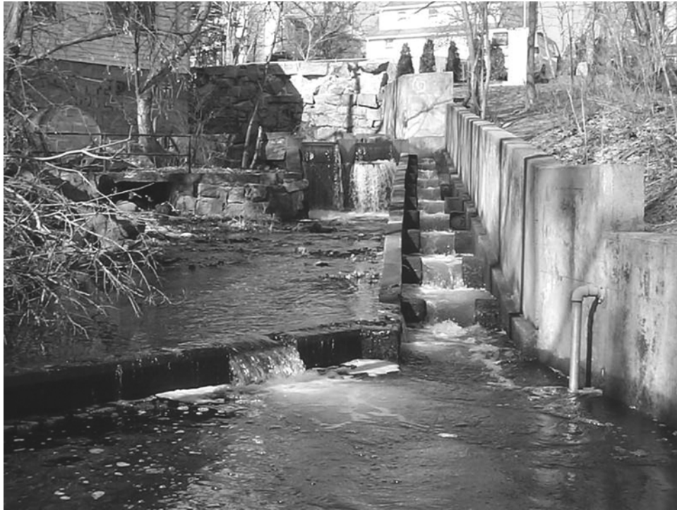
Fish ladder above USGS streamflow gaging station at outlet to Whitmans Pond in East Weymouth, MA, 01105608.
