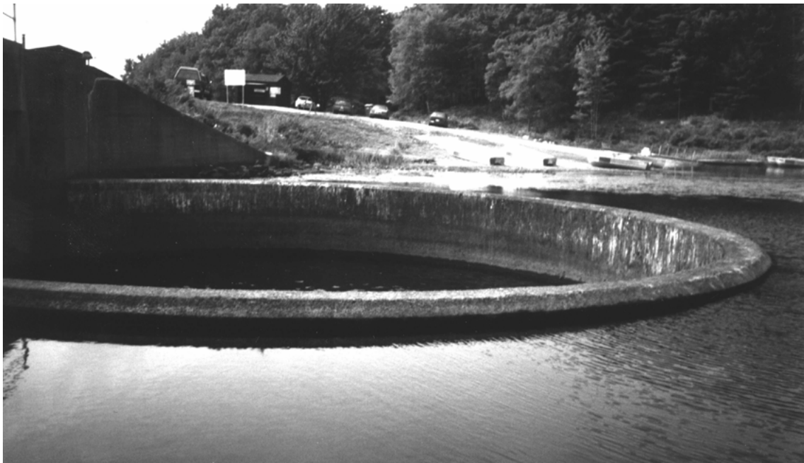
Horseshoe weir showing no flow into Quabbin Reservoir, Sept. 14, 1995, East Branch Swift River near Hardwick, Mass. (photo by L. Y. Comeau).
