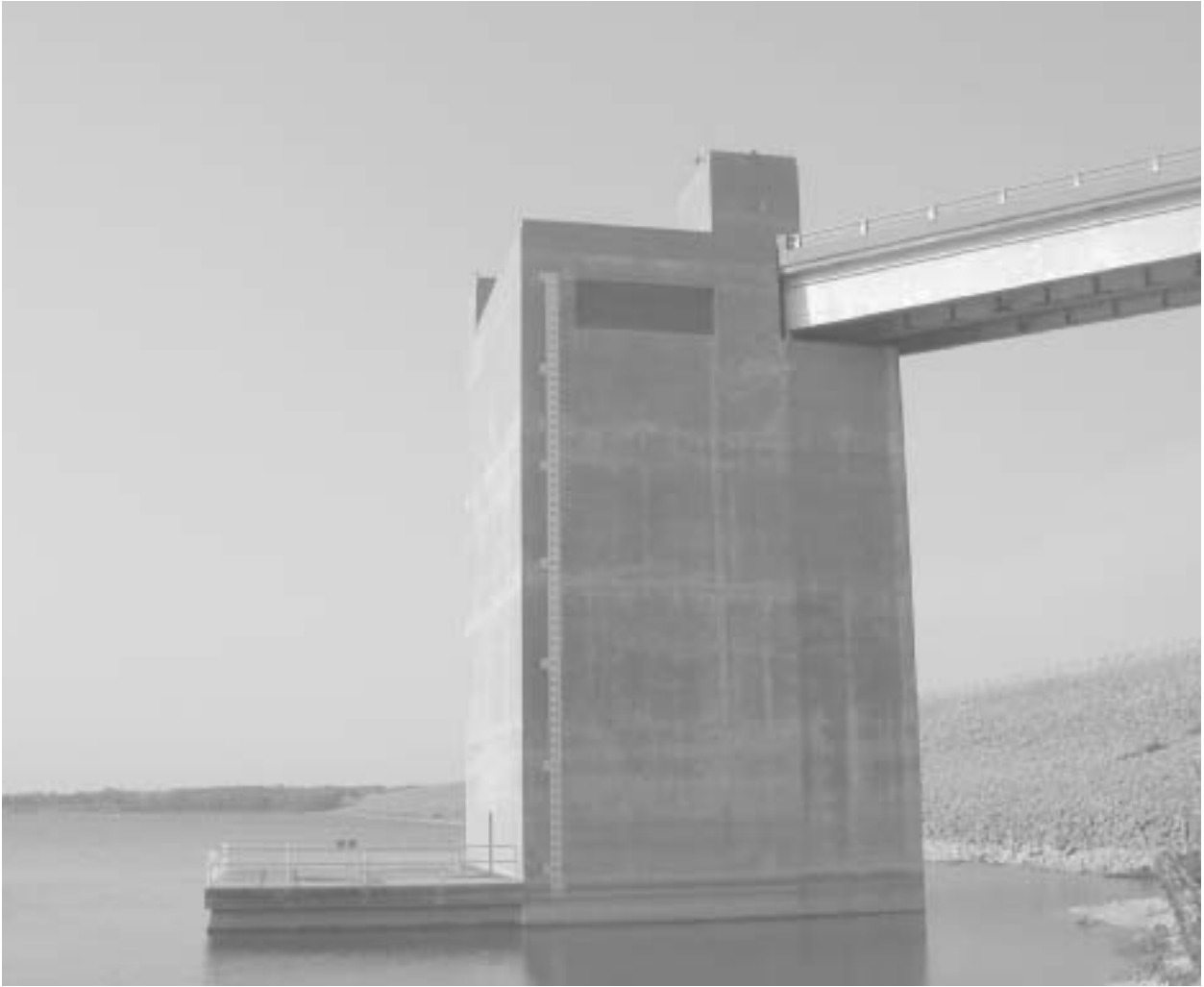
Control tower at Milford Lake near Junction City, July 16, 2003. Lake elevation near conservation pool, 1,144.84 feet. Photograph courtesy of D.D. Wilmes.
