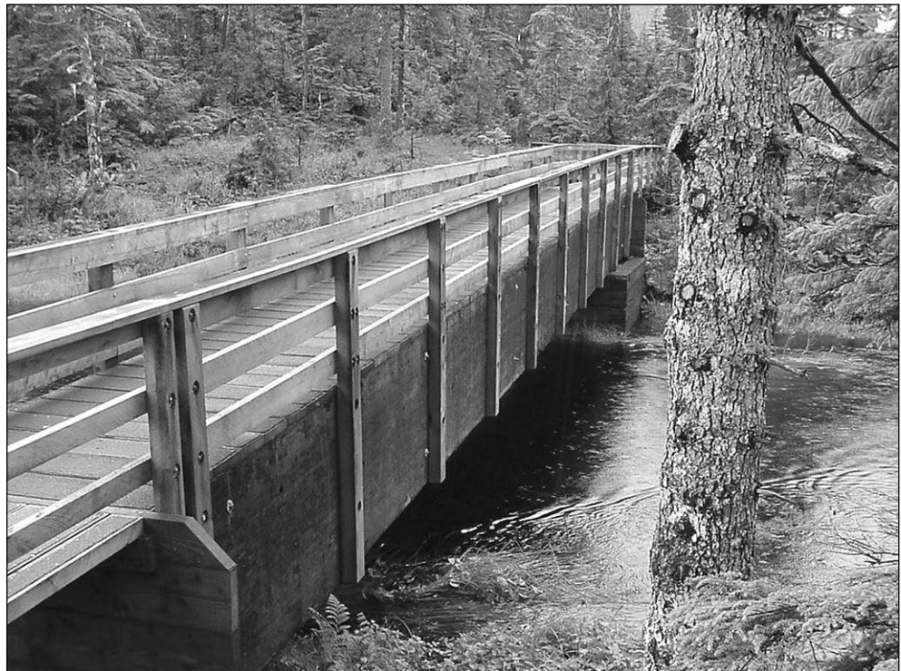
Figure 3—Tongass National Forest wood bridge.
