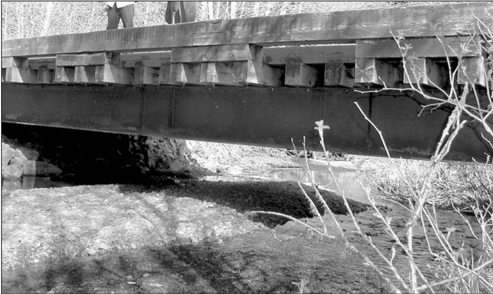
Figure 4—Tongass National Forest wood deck on steel superstructure.
