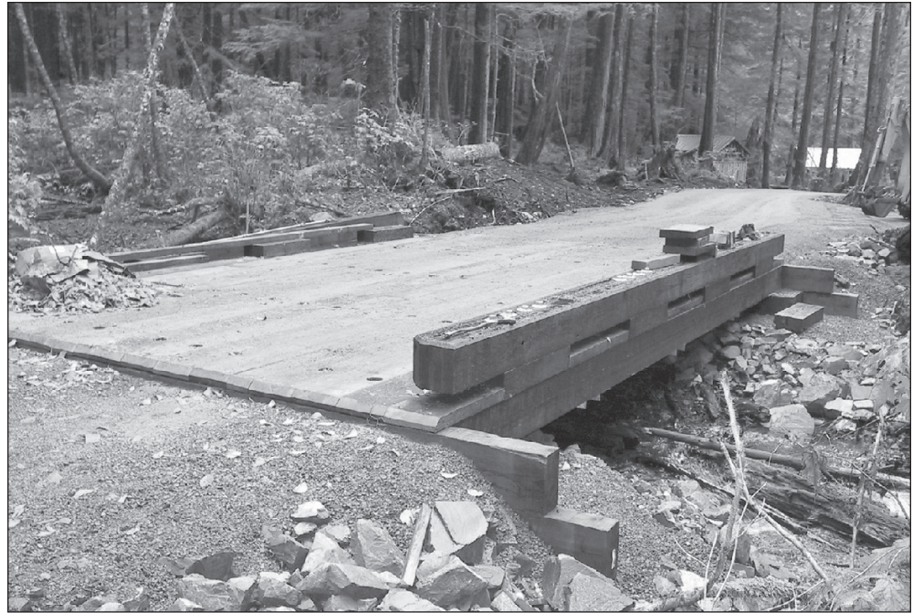
Figure 6—Tongass National Forest wood utility bridge.
