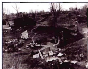
Dorothea Lange Migrant workers' camp, outskirts of Marysville, California. The new migratory camps being built by the Resettlement Administration will remove people from unsatisfactory living conditions such as these and substitute at least the minimum of comfort and sanitation. April 1935
