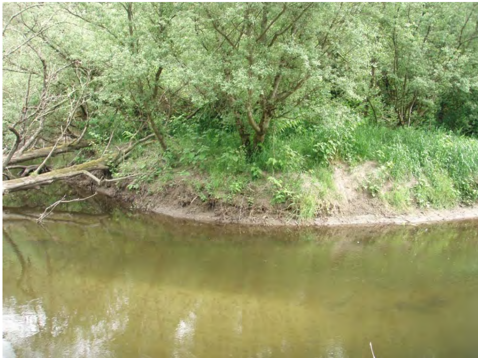
Riverbank on Soos Creek May 2007 near Logjam
