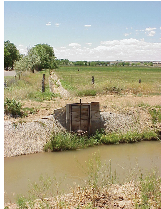
The headgate of an acequia (or ditch) near Paseo del Norte in northern Albuquerque.
