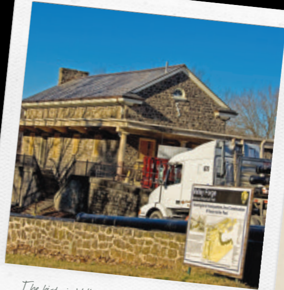
The historic Valley Forge Train Station is being restored to serve as a point of orientation for visitors to Washington's Headquarters.
