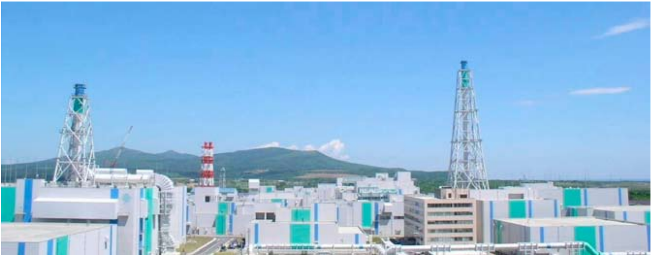
▲ Rokkasho Reprocessing Plant
