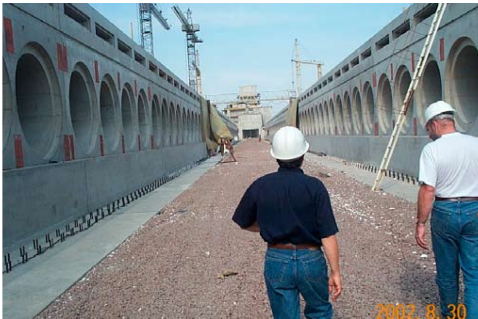
▲ Spent Fuel Storage
