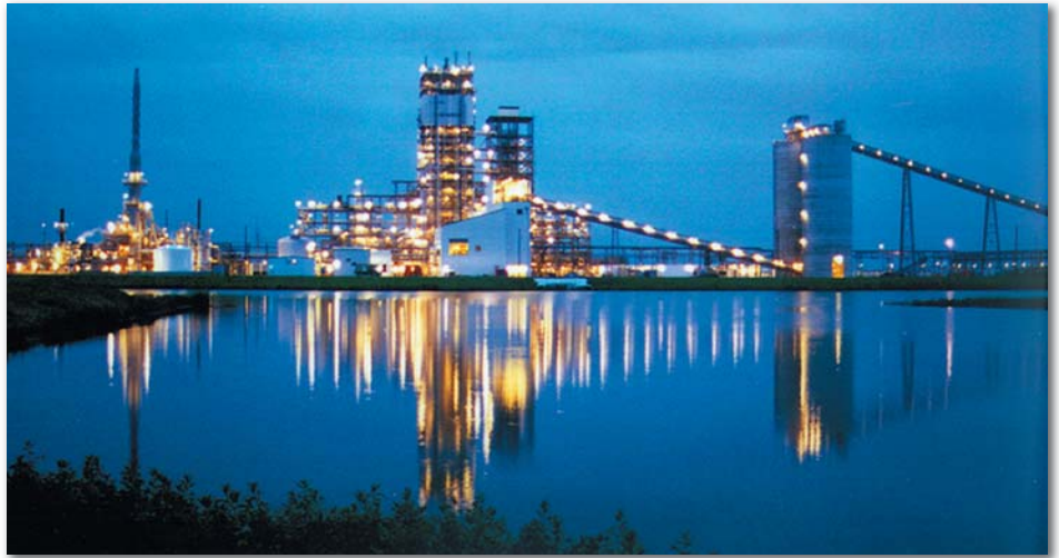
Tampa Electric's Polk Power Station
