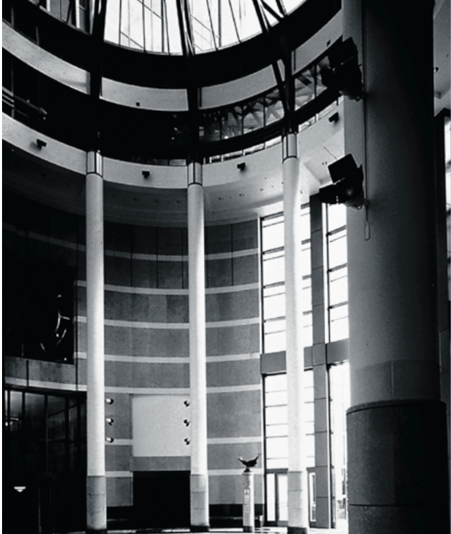
Oakland Federal Building, Oakland, CA
