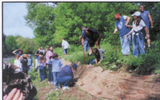
Winchester Elementary students and West Seneca AmeriCorps planting bare-root seedlings through Geo-jute erosion control fabric, Spring 2001.
