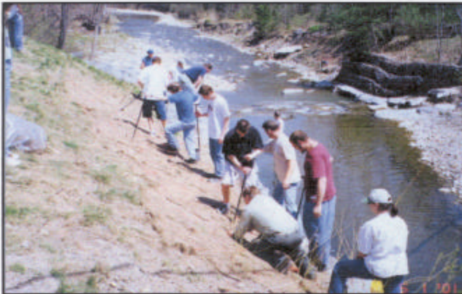
Holland High students and Erie County Department of Environment & Planning and USDA Natural Resources Conservation Service volunteers planting Red osier dogwood and Streamco willow bare-root seedlings through Geo-jute erosion control fabric, Spring 2001.
