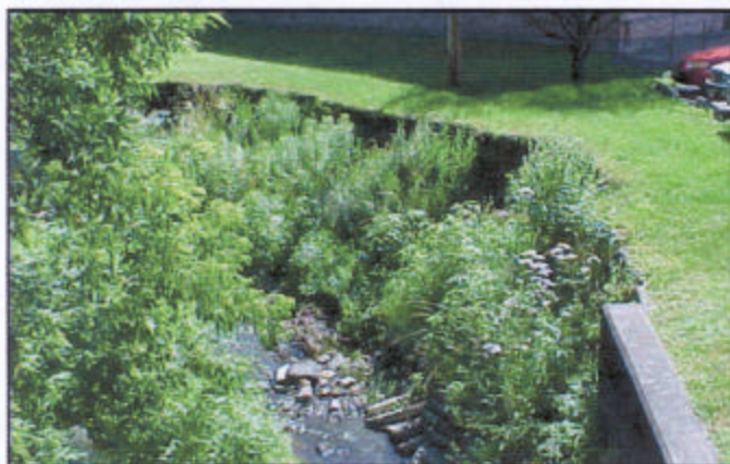
Streambank before treatment, Summer 2000.
