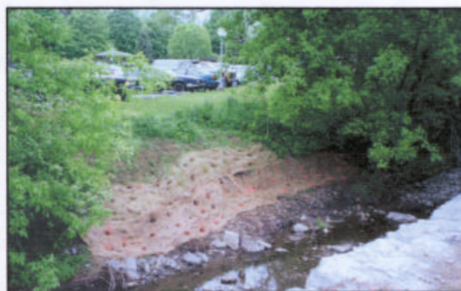
Finished bank opposite rock wall planted with Red osier dogwood and Streamco willow bare-root seedlings through Geo-jute erosion control fabric, Spring 2001.
