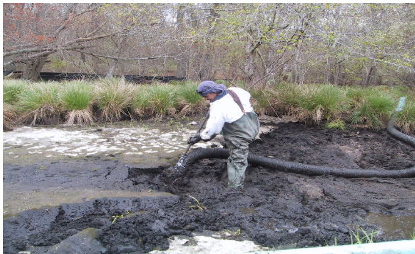
Photograph 1. Sediment removal using a vacuum guzzler
