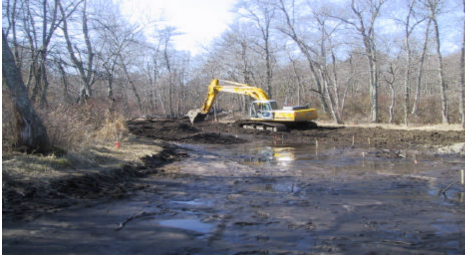
Photograph 2. Sediment removal using a long-arm excavator
