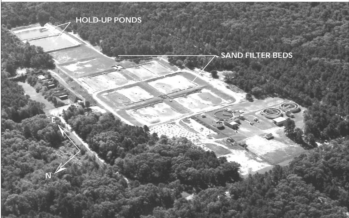
BNL's sewage treatment plant contains eight sand filter beds and surrounding sand berms. Isolated areas will be excavated to remove contamination.
