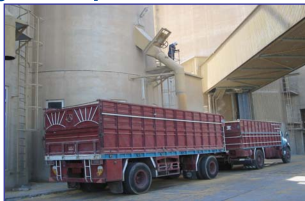
A recent shipment of grain to Umm Qasr port is being loaded onto trucks for delivery after being transferred into the newly restored grain silos. (Bechtel Photograph)
