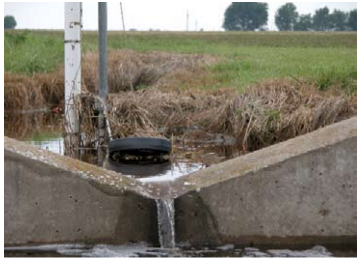
An instrumented water weir used to measure water runoff.
