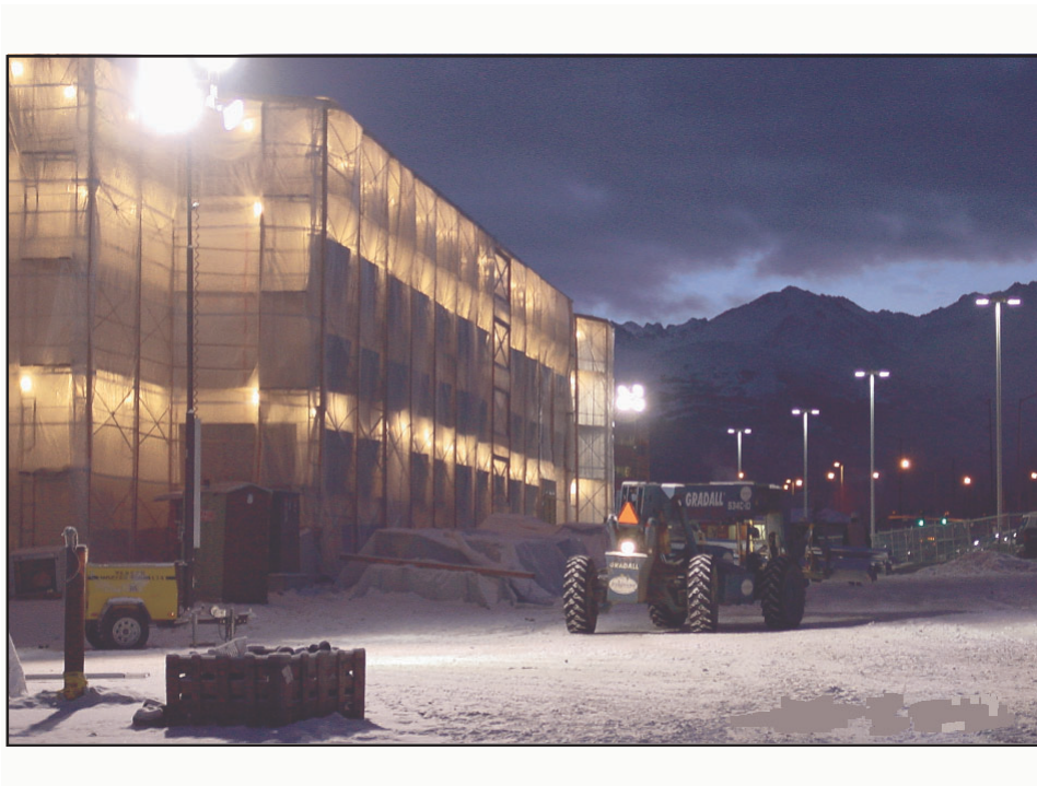
Photo 21: Cold weather construction site in Anchorage, Alaska
