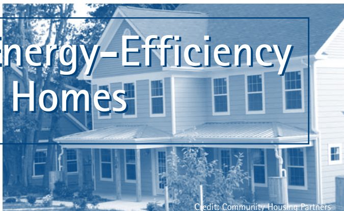
Credit: Community Housing Partners
