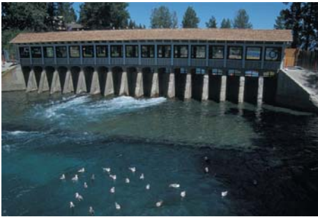
Lake Tahoe Dam
