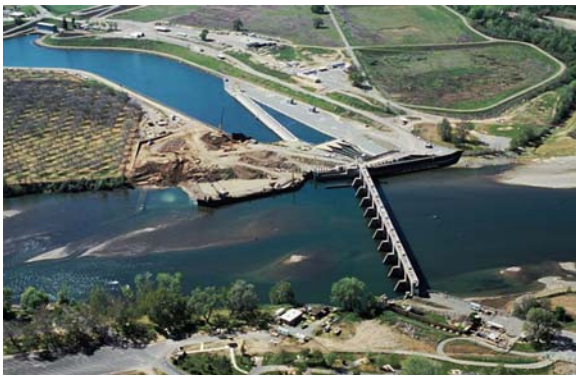
Red Bluff Diversion Dam
