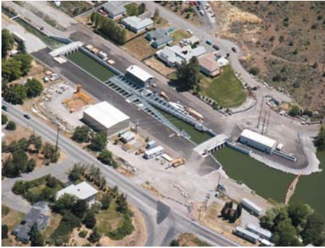
Aerial view of the "A" canal fish screen and associated facilities.
