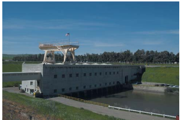
Tracy Pumping Plant
