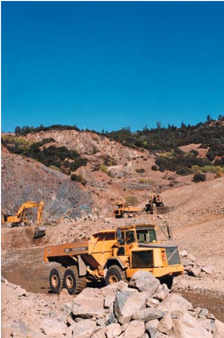
Construction of the American River Pump Station Project underway in 2004.
