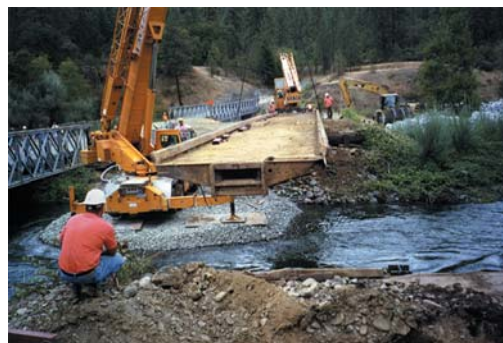
Trinity River Bridge construction in 2004.
