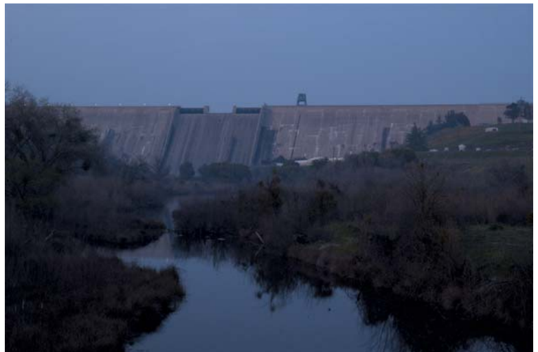
Lower San Joaquin River near Friant Dam
