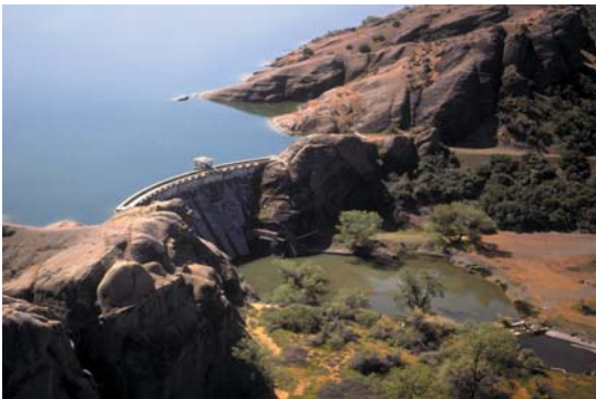
East Park Dam and Reservoir
