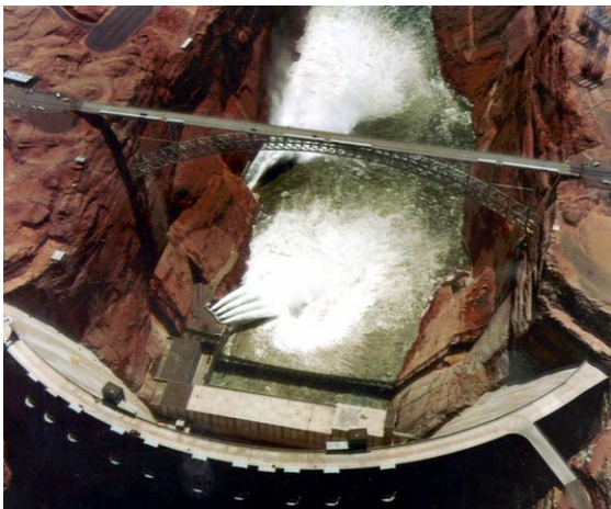
Figure 1. Aerial view of Glen Canyon Dam, Arizona.
