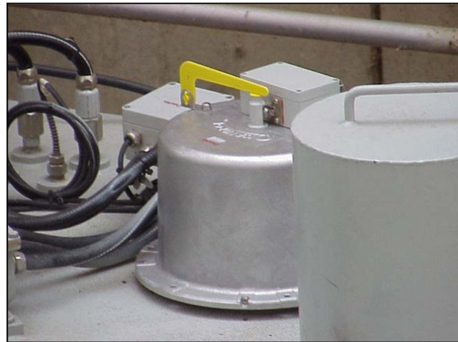
Figure 10.— Pressure Relief Device.
