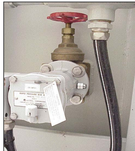
Figure 12.—Sudden Pressure Relay.
