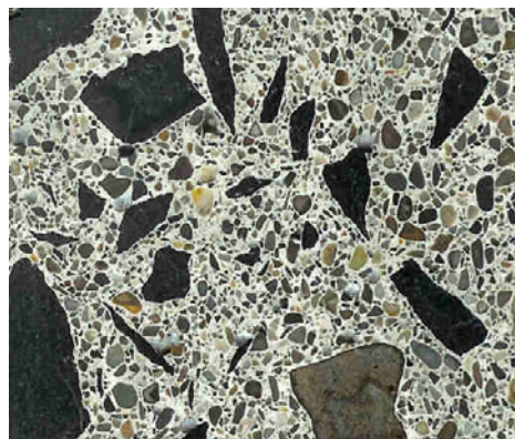
Figure 14. Polished sample of concrete from the Monroe Street Bridge in Spokane, Wash., showing reaction rims on andesitic aggregate particle and on smaller aggregate particles, indicating reaction with alkalis in concrete.
