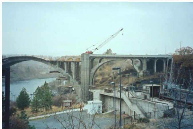
Figure 12. Monroe Street Bridge in Spokane, Wash., undergoing rehabilitation work in fall 2003.
