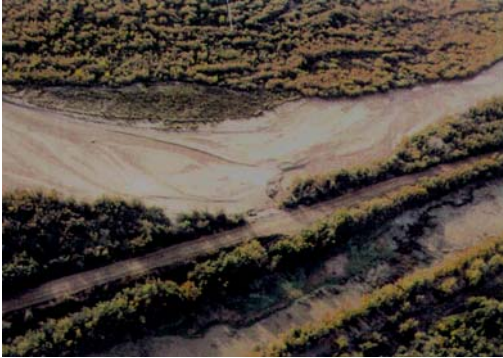
Figure 1.1 Levee Breach in 1991 as a Result of the Sediment Plug
