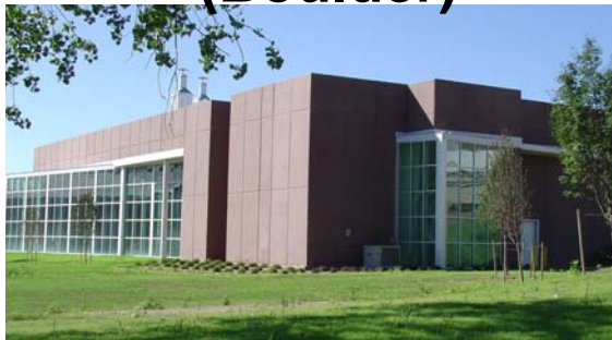
Central Utility Plant (Boulder)
