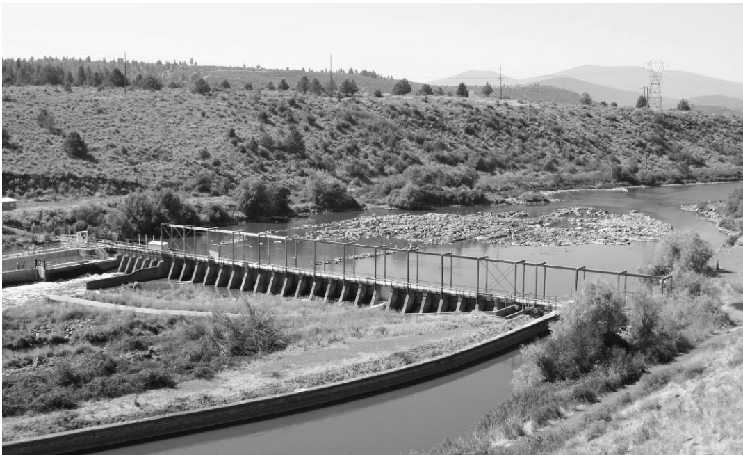
Figure 2. Photo of Link River Dam. Spill gates and fishway are on the far left and the Eastside hydropower bay on the right side. The reef is upstream of the dam. The two channels that were blasted through the reef are located on each side of the reef near the shoreline.
