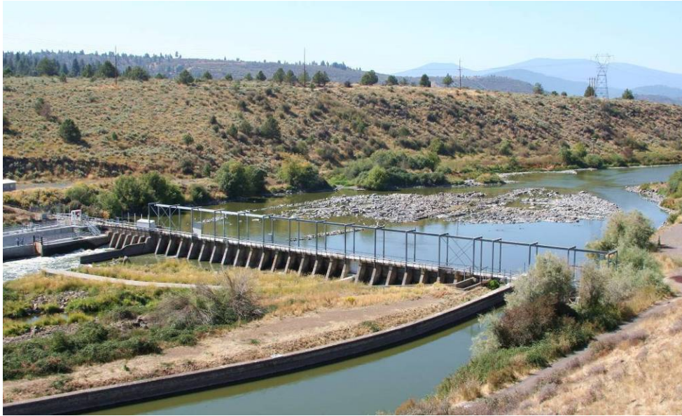
Figure 3-10. Photo of Link River Dam looking upstream. Spillway and fish ladder (fishway) are on the far left and the Eastside hydropower bay on the right side foreground. The reef is upstream of the dam. The two channels that were blasted through the reef are located on each side of the reef near the shoreline.
