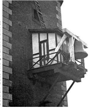
Fog bell on the side of the fort.
