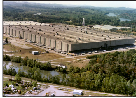
Indoor PCAT location: Building K-33, East Tennessee Technology Park
