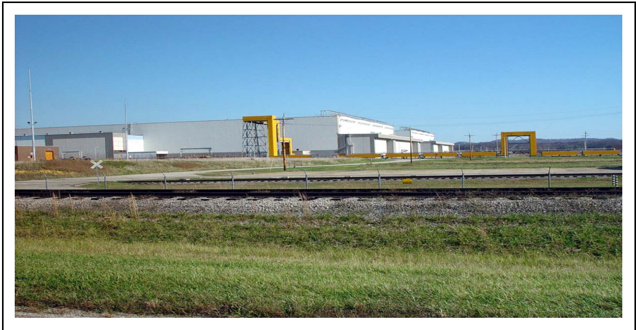
Figure 3-6 View of the X-3001 and X-3002 Process Buildings [Looking Northeast] (USEC, 2005)
