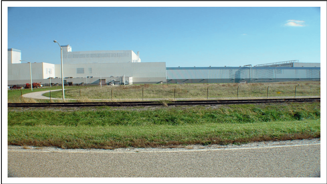
Figure 3-4 View of the X-7725 and X-7727H Facilities [Looking East] (USEC, 2005)
