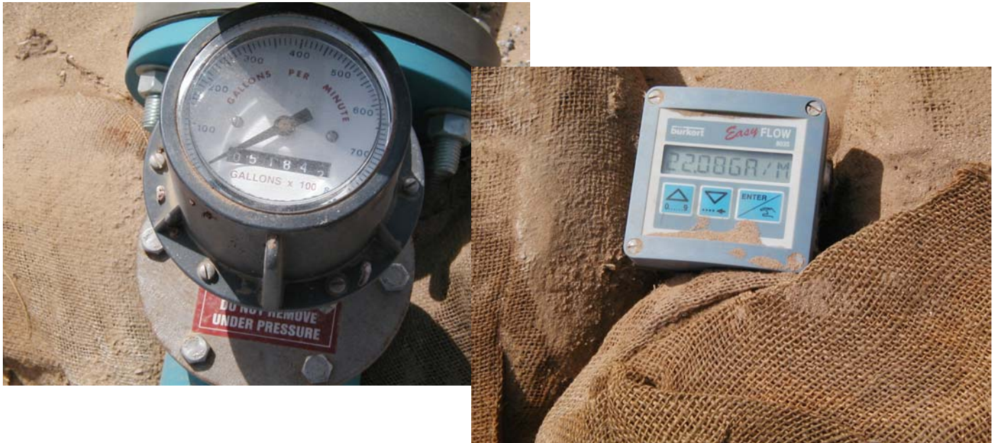
Figure 3.4—Metering of flow from Sea intake and between ponds.
