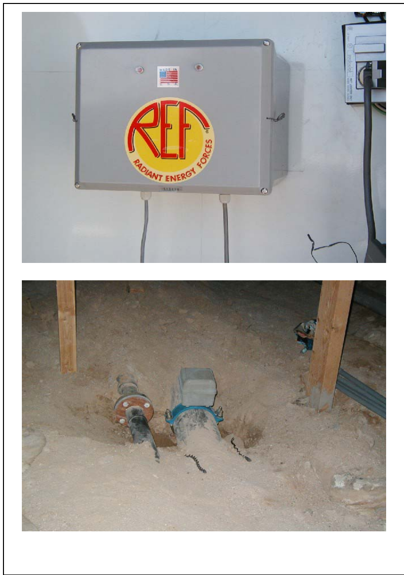
Figure 5.11—REF barnacle removal system.
