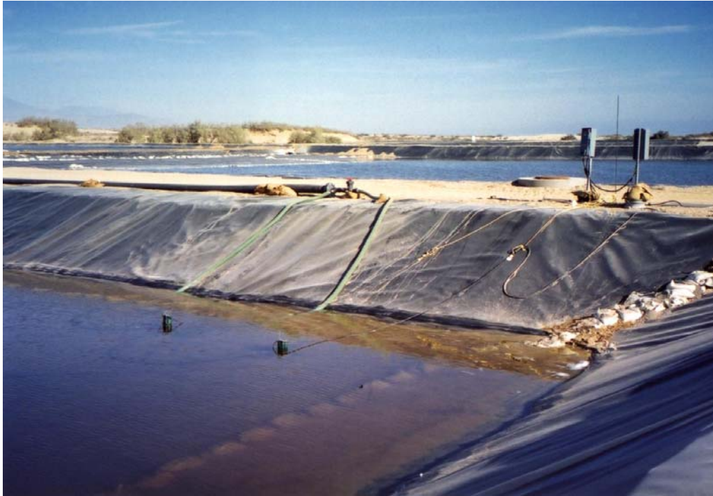
Figure 3.2—Pumping between major ponds.
