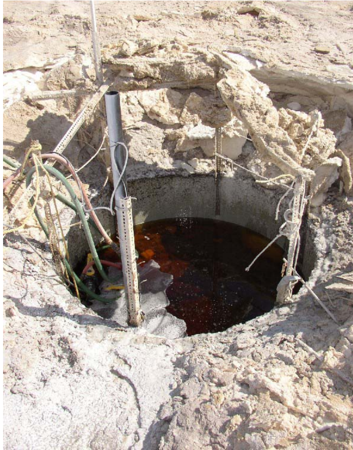
Figure 5.4—Sump used to drain and pump entrained brines
