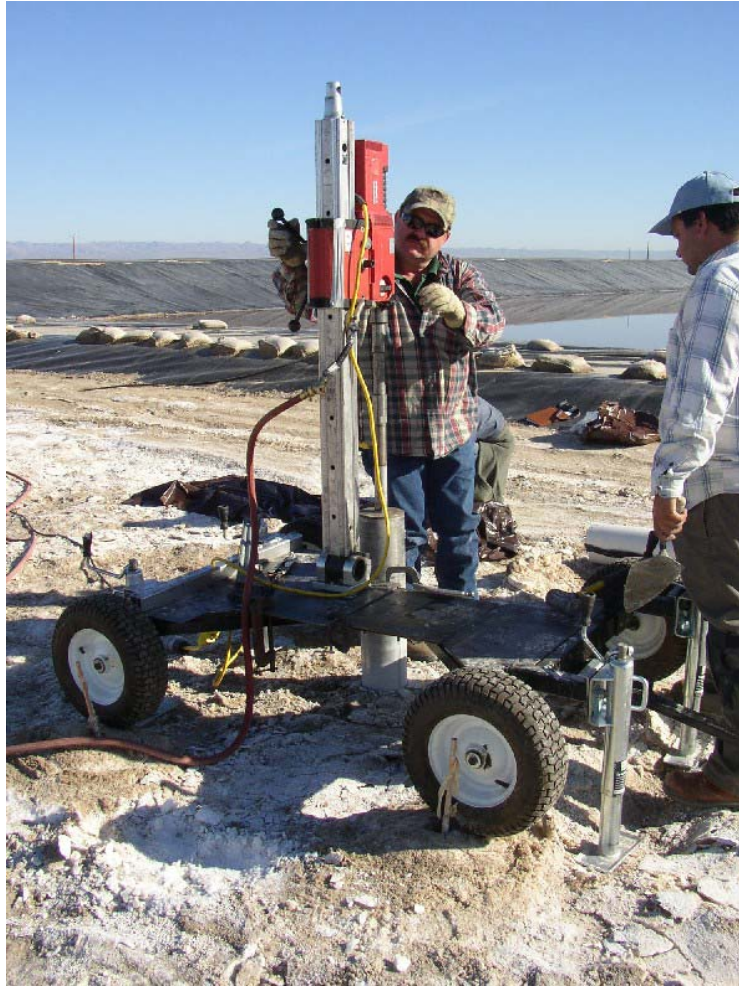
Figure 3.14—Core drill and platform.
