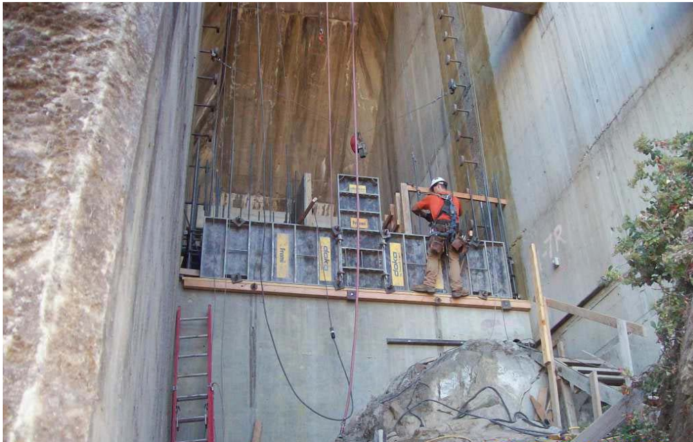
A worker installs a diaphragm wall form for a concrete placement.
