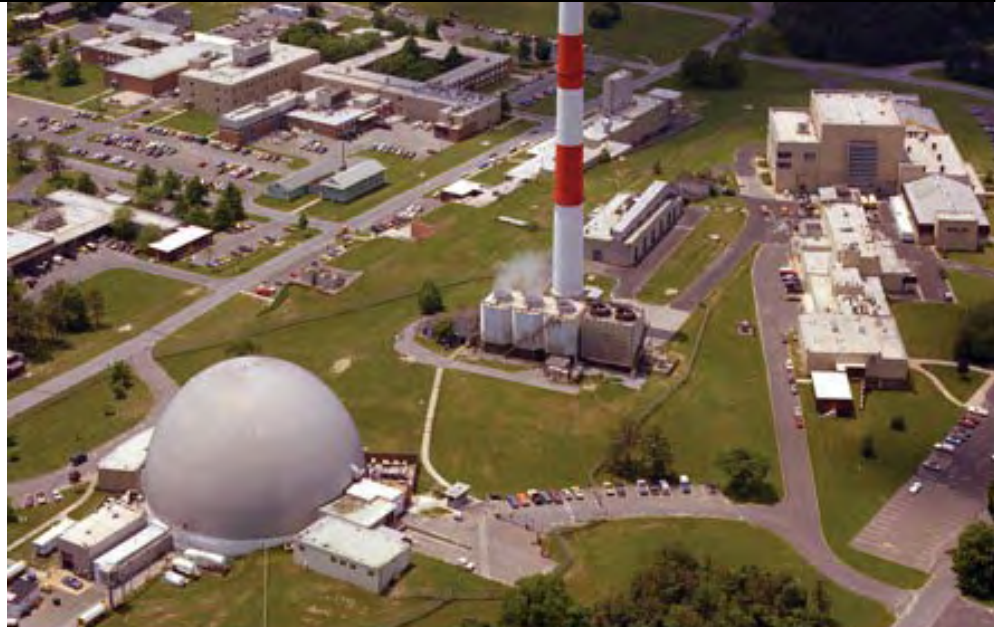
Operating from 1965 to 1996, the High Flux Beam Reactor (domed complex, bottom left) was constructed solely for scientific research, providing neutrons for materials science, chemistry, biology, and physics experiments.
